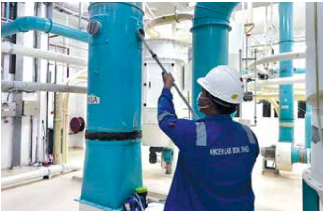
Stack Emission Monitoring
