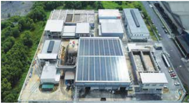
Solar Panel on the roof top of the Primary Processing Plant
