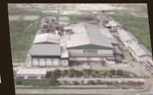
DPP Processing Plant at Sitiawan, Perak
