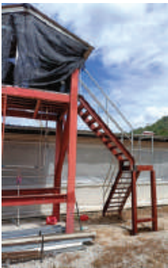
Installing staircase inside breeder farm
